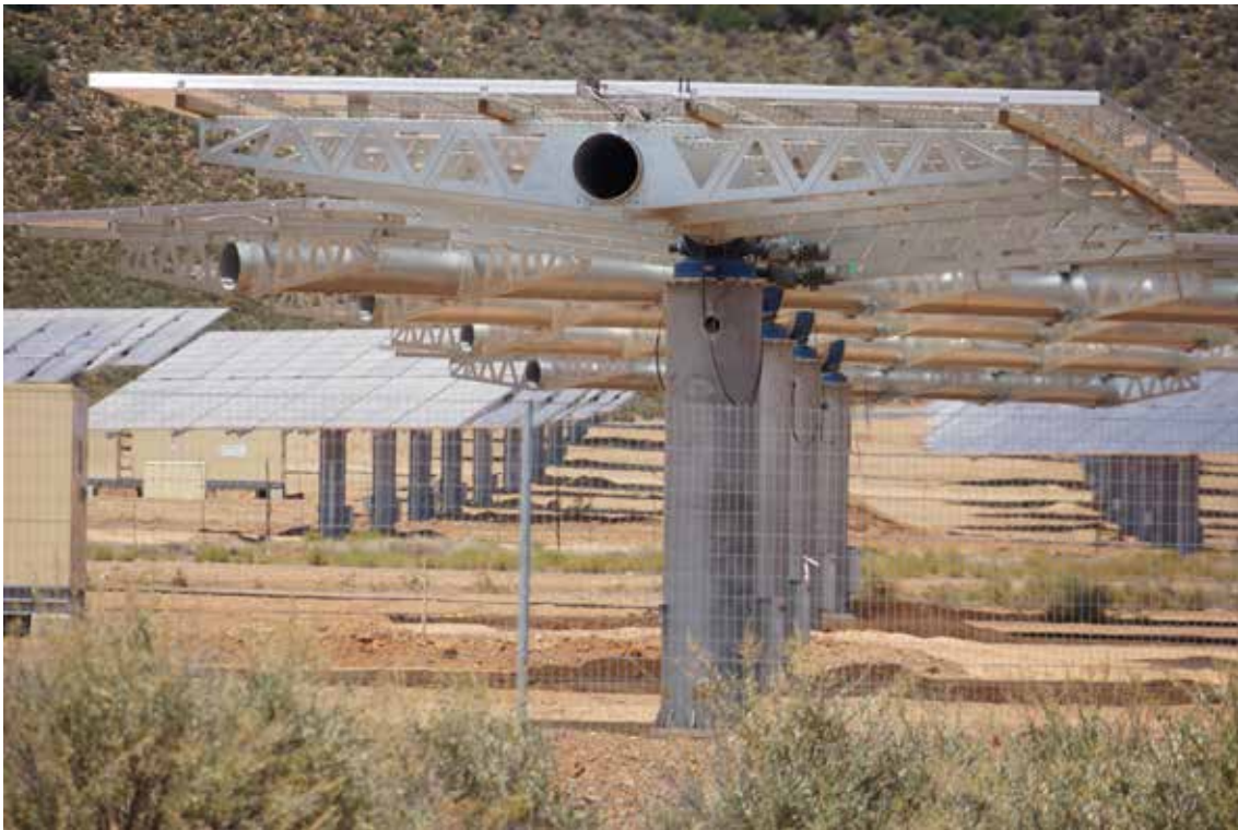
Solar trackers during construction of the solar farm at Touws River
