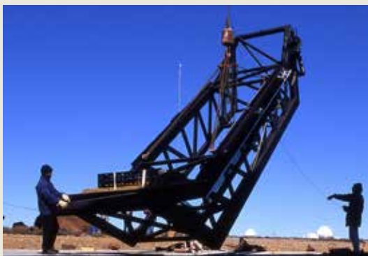
Lifting the tracker beam
