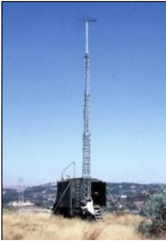
Figure 5: UHF Foliage Penetration Radar Test Facility.
